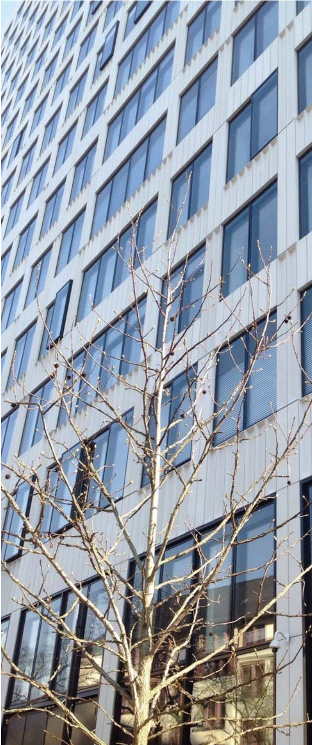
Around 13,000m 2 GRC units were used in the refurbishment.
