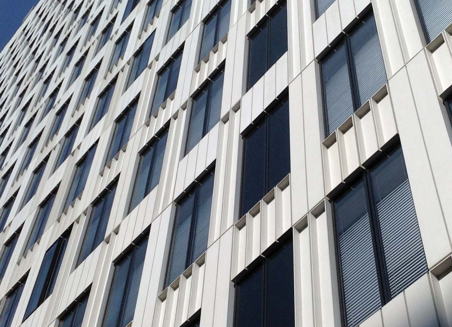
The LEO in Frankfurt, formerly known as Poseidon House, has been clad in glass-fibre-reinforced concrete.
